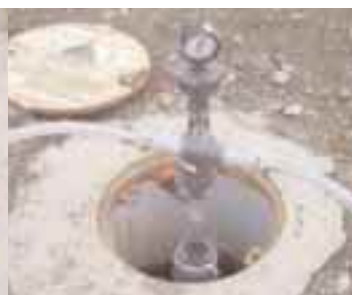
Sulfuric acid injection in progress
