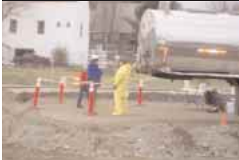
Containment trench around tankers
